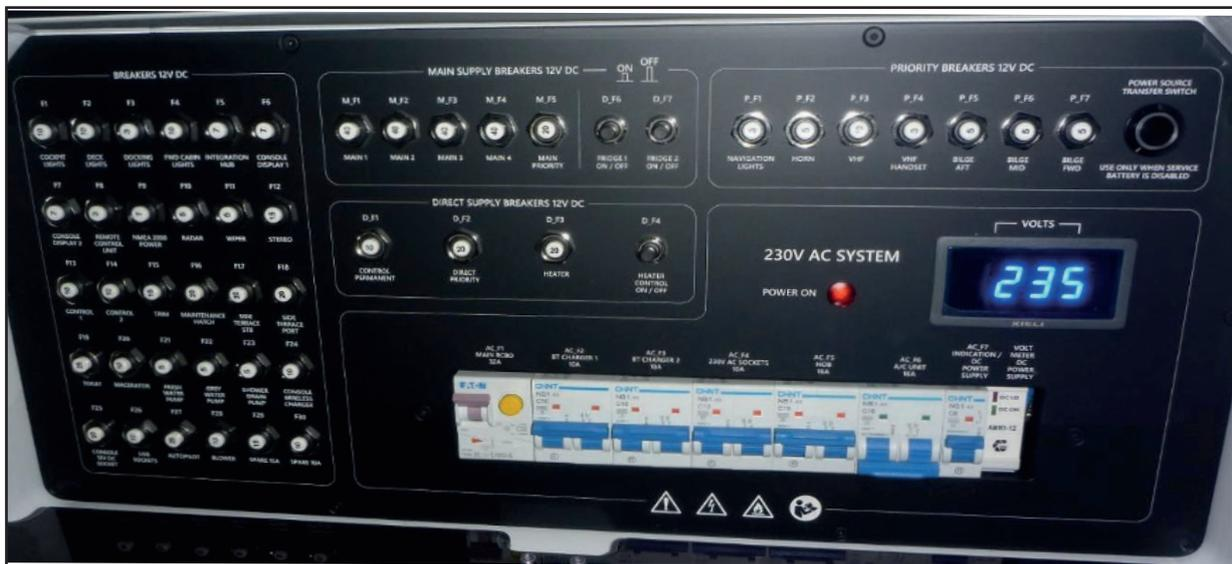
12V DC circuit breakers and 230 V panel board
